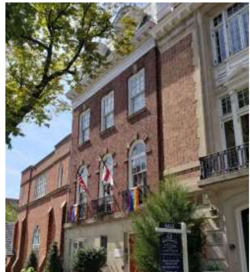
PLATE 2-45: St. Margaret's Episcopal Church, 1830 Connecticut Avenue, NW (Louis Berger photo, 2019)
